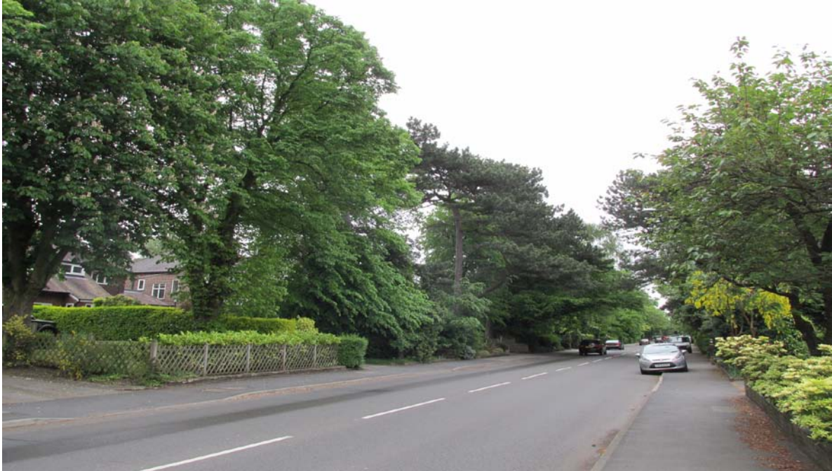
Image above shows distance view down Brooklands Rd including Pine and Lime tree in front garden of 297 Brooklands Rd
